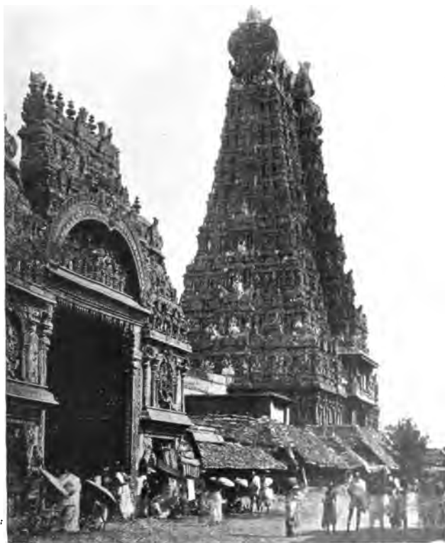
MADURA — GRAND GOPURA
